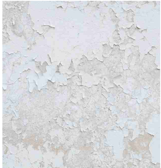
Acrylic Paints weather and deteriorate due to atmospheric influences such as UV, rain, pollution and require repainting every 5 - 10 years.
